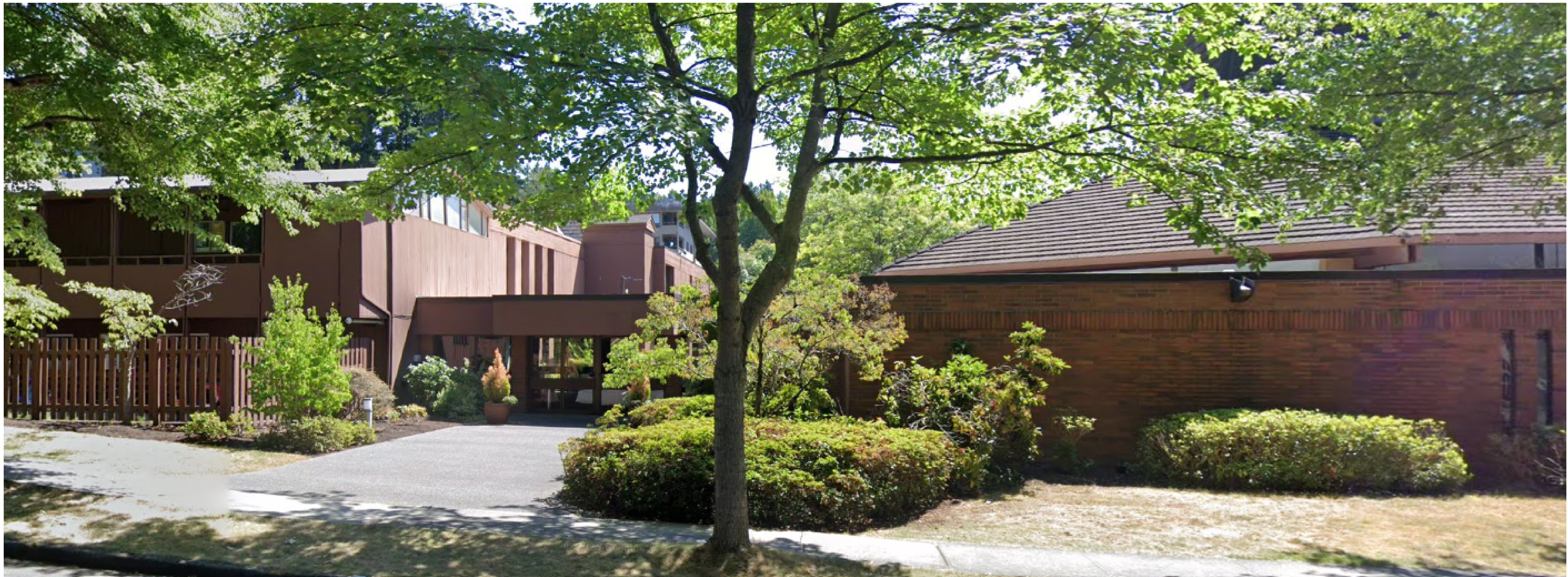
NORTHERN STREET VIEW - FACING NORTH PART OF NARTHEX, SANCTUARY, AND PATIO
