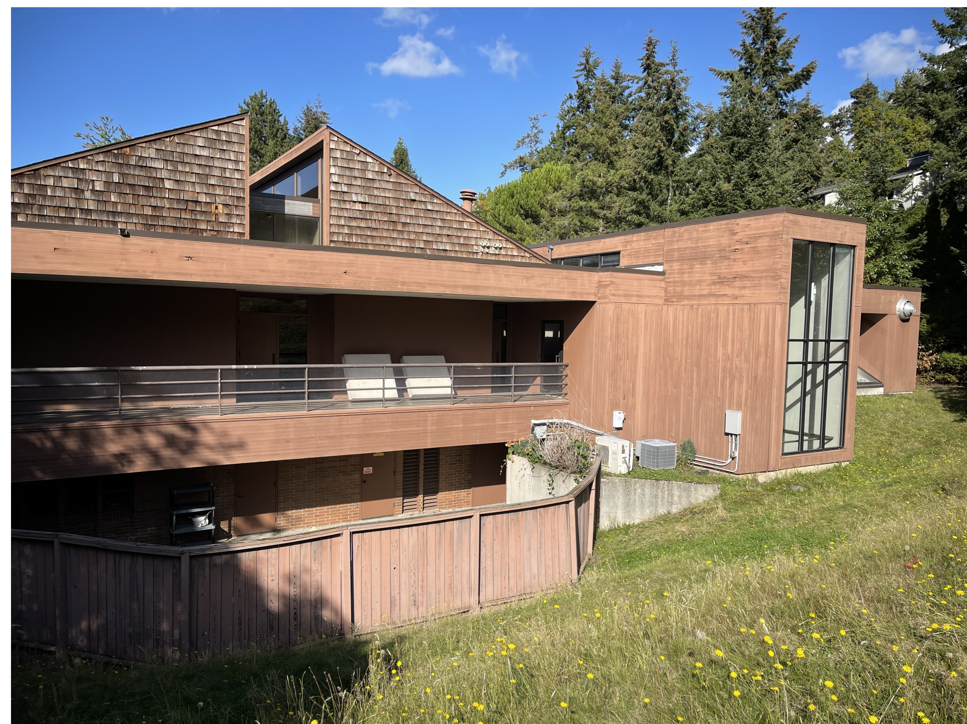
WESTERN VIEW - FACING SECOND FLOOR CLASSROOM SPACES AND PATIO
